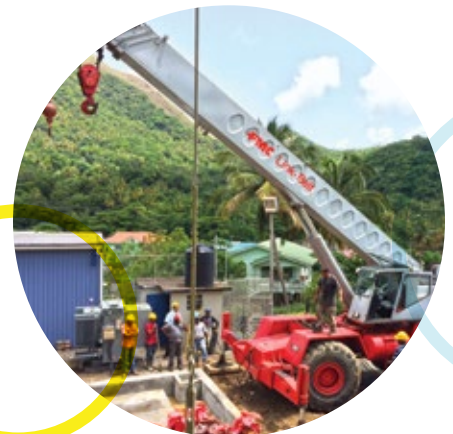
The Soufriere substation was re-commissioned following its shut down in May 2012. Work at the site involved replacing the damaged transformer and upgrading the protection system at the facility
